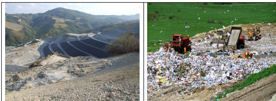
Figure 4. Controlled landfill is safe stockage of solid waste with confinement in a suitable waterproofed area, minimizing the risks for man and the environment. Anaerobic processes of decomposition of organic materials can be contained with the production of biogas and leachate.
