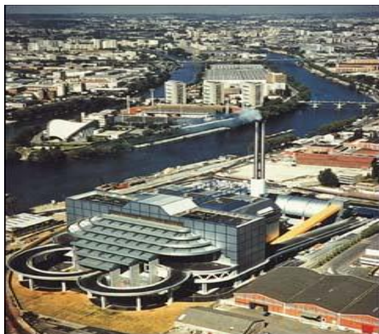
In Paris, France, the Compagnie Parisienne de Chauffage Urbain supplies several thousand homes with hot water from incinerators located on the outskirts of the French capital
