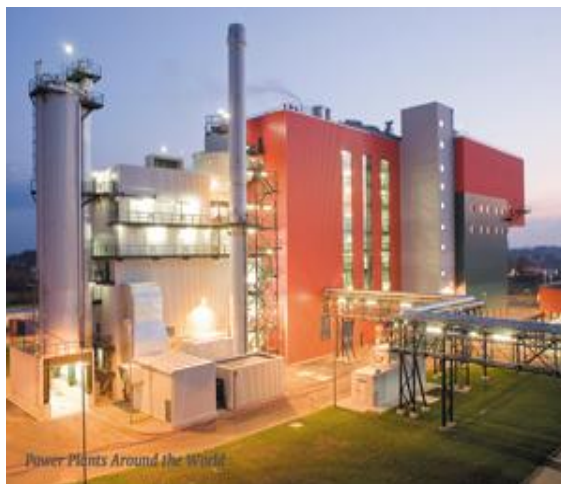
Incinerator MSW, Premnitz, energy from waste [operator EEW, Germany, 2009, cost 70 million euros]
