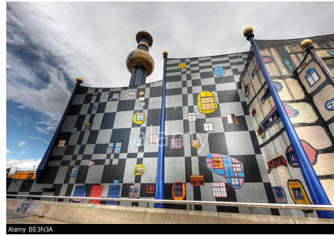
Figure 7. The Spittelau waste incineration plant processes around 250,000 tones of MSW every year. [The incineration plant produces approximately: 40,000 MWh of electricity, 470,000 MWh of district heating, 6,000 tones of scrap iron, 60,000 tones of clinker, ash and filter cake. The environmentally friendly heating produced at Spittelau is enough to heat 60,000 households in Vienna in a year.
